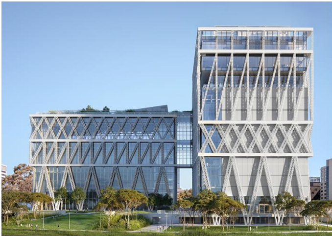
Powerhouse Parramatta (Under construction)
