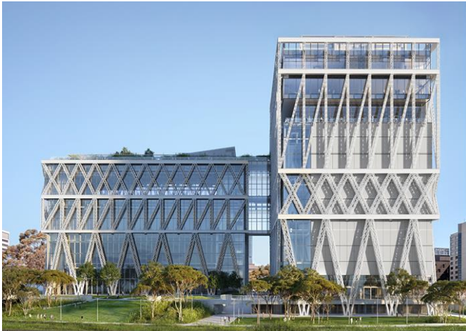
Powerhouse Parramatta (Under construction)
