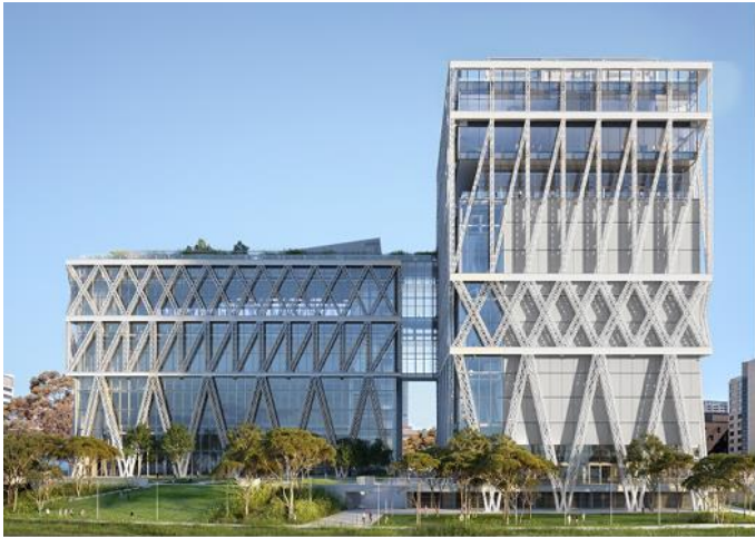
Powerhouse Parramatta (under construction)
