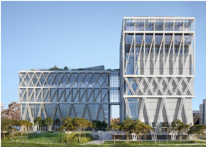
Powerhouse Parramatta (Under construction)
